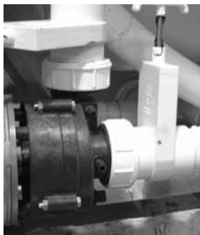
Slice Valve and Pump Union
