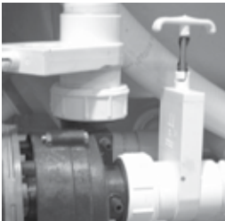
Slice Valve and Pump Union
